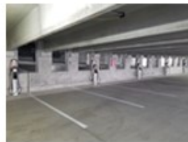
Lincoln Square—new multi-unit housing complex on Broad Street, Philadelphia—installed 13 Electric Vehicle Charging Stations in the state of the art "GREEN GARAGE"
