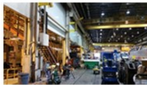
We installed the electrical infrastructure related to the Fall Protection System located at the NJT Meadowlands Maintenance Complex
