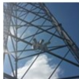
We installed state of the art perimeter protection via a Fiber Optic Detection System at one of many cell towers
