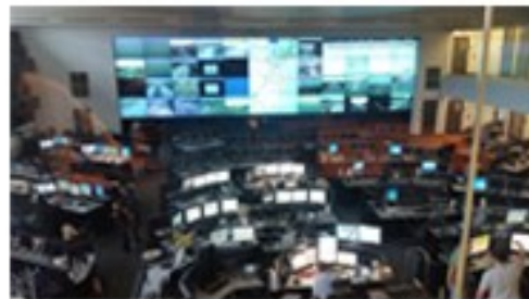
Completed electrical and IT wiring overhaul at the Statewide Traffic Management Center (STMC) occupied by the NJTA, DOT, NJSP, & GSP
